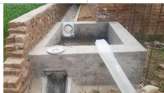
Picture 4.7: Balyala: Plastic foldable pipes being used for irrigation before lining of watercourse
