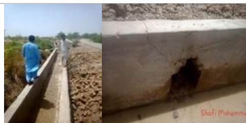
Picture 4.107: View of Watercourse with Damaged Portion, Sohbatpur, Balochistan
